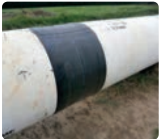
Insulation of welded joint on pipe with 3LPP insulation
