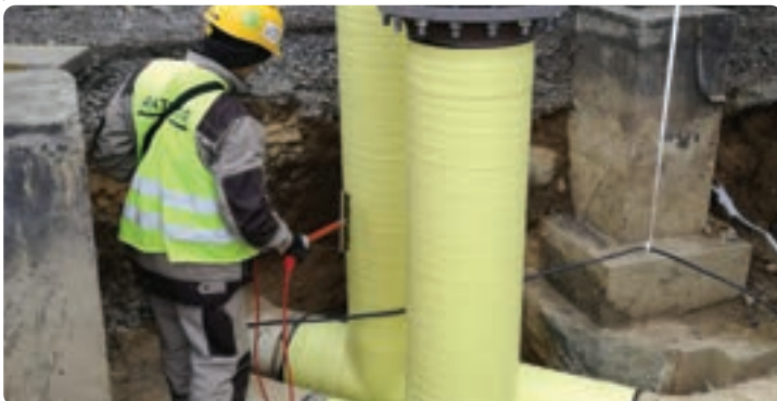
Checking the tightness of the coating with a spark flaw detector
