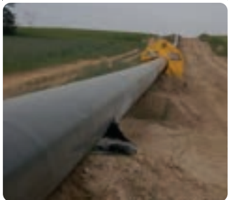
Pipeline DN 700 isolated by ANTICORRay® WSS60 heat shrink sleeve
