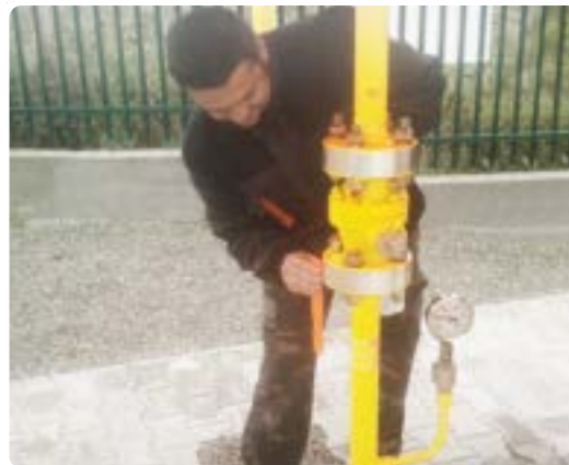
Insulation of a flange joint
