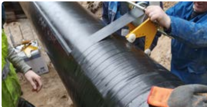
Application of corrosion protection coatings on pipelines
