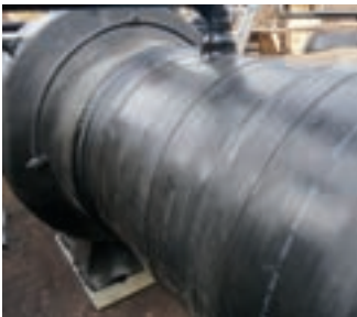
Insulation of welded joints on the valve DN 1000
